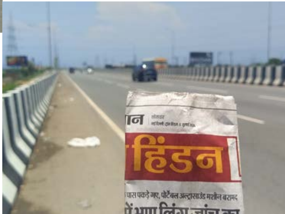
Sabli Overbridge Hapur Bypass fc Moradabad 30x15
